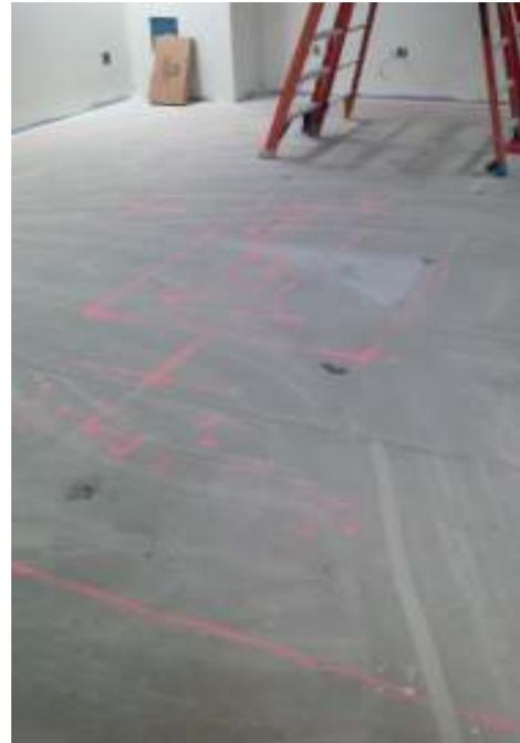
**Figure 2:** Mock-Up Process of Operating Room
